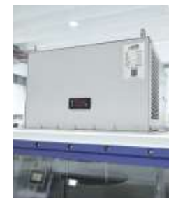
Air conditioner for electrical control box
